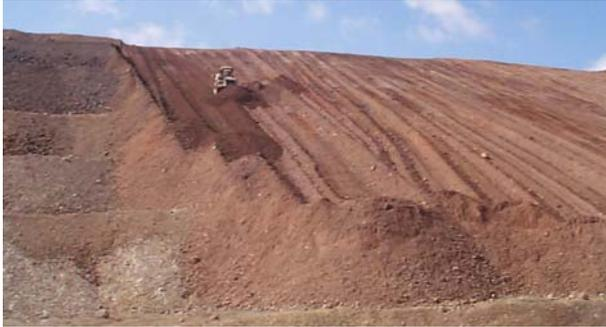
**FIGURE 7** Heap Leach Pad Side Slope Contouring.
