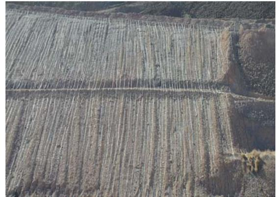
**FIGURE 9** Side Slope Emitter Placements.
